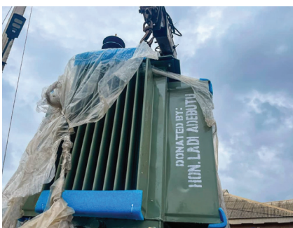
DELIVERED TO SITE
