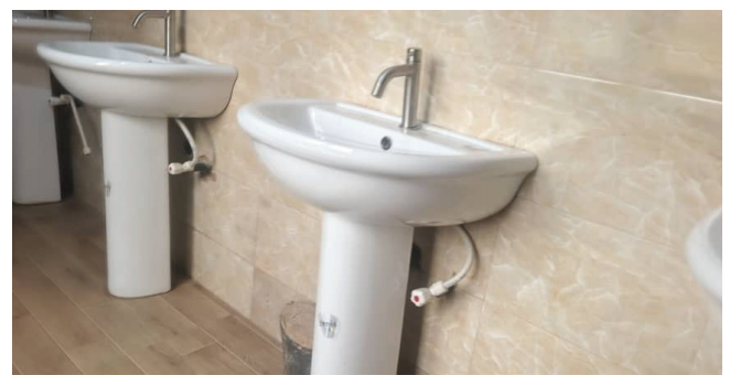
NEW SANITARY FACILITIES
