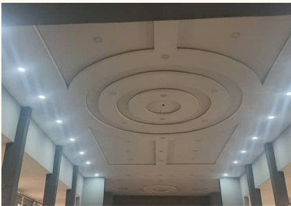
NEW CEILING & LIGHTING
