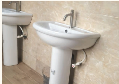
NEW SANITARY FACILITIES
