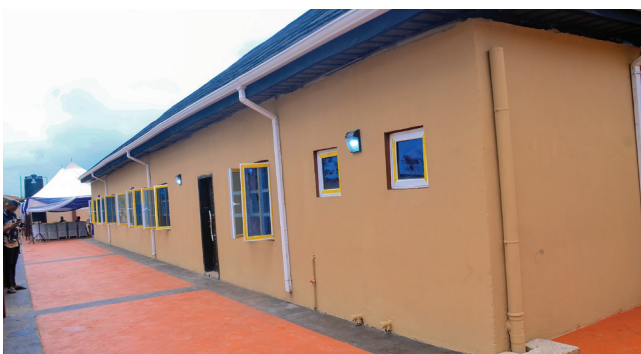
THE COURTYARD, COMPLETED
